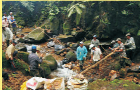
The dam built by village volunteers to run the micro-hydro turbine
