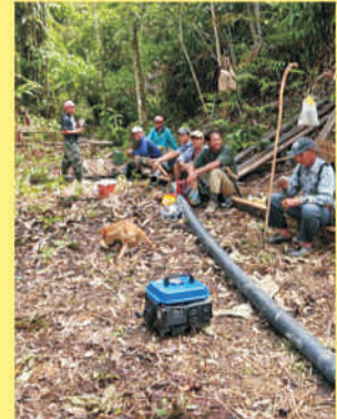
Laying of HDP pipes from dam to turbine shed
