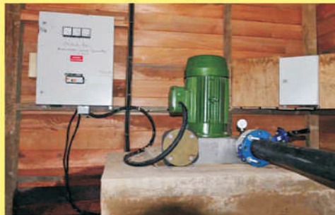
Micro hydro turbine & control panel in the shed
