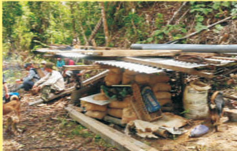
Roofing sheets, cement & timber arrive safely
