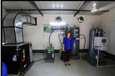
GG 212746 provided funding for the purchase of Medical Oxygen Supply System for Ispat Hospital in Kolkata. The Oxygen generation system can fill up Oxygen cylinders when needed as well as provide direct oxygen supply to patients in hospital wards. Supply is 24x7 and machines have a 5 years minimum lifespan and require minimal maintenance. The GG also provided funding for a purchase of a Ventilator for the same Hospital. DG D3310 Dolly Yeap (above) is seen inspecting the Oxygen Plant and Ventilator. Dr. Shahul and Mrs. Michelle Hameed as well as Director Peter and Mrs. Tanya Brock accompanied DG Dolly for this visit to Kolkata on 8 March 2022. Special thanks to PP Terry Chun and PP Frank Yih from RC Shanghai and Hua Qiao Foundation for their unstinting support for this Project.
